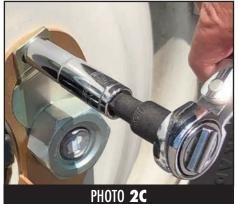
**Step 2.** Installing Bracket Locking Tabs
