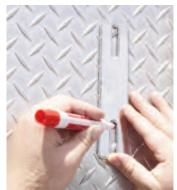
**3. Mark** Mark the center point in both openings of the back plate.
