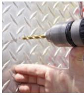
**4. Drill** Using a 7/32" drill bit, drill completely through marked positions.
