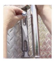
5. Insert Bolts Insert bolts with washer through flagpole holder mounting bracket and through previously drilled holes. Note: Remove any protective PVC coating from mounting bracket.
