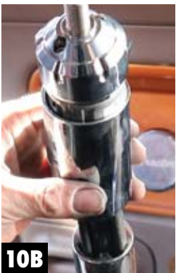
Step 10 Slide Up the Base Cover • Slide up the base shift cover (See Fig. 10A & 10B). Install the 2 Torx T20 screws that were taken out of the old base cover (10C).
